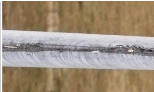
Example 2: Leading edge erosion, CAT 3 Repair cost: €2,000
