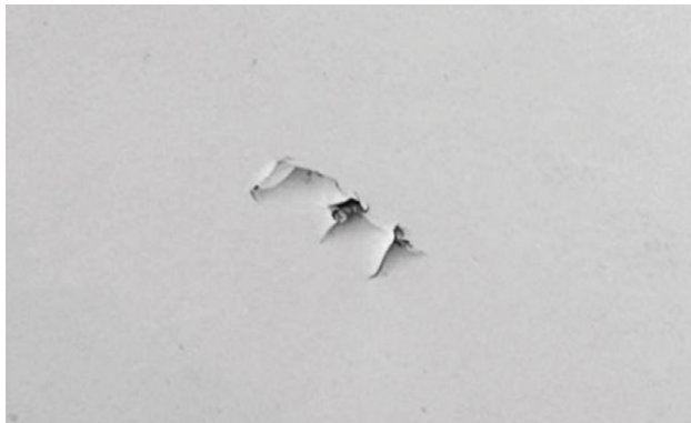
Example 1: CAT 3 Crack near root Repair cost: €2,000
